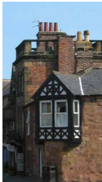
Dormer windows, bay windows, balconies, gables, chimneys are all shown here as more elaborate
