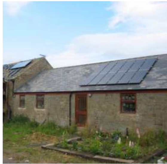
Photovoltaic panel insertion into the roof of an old cottage
