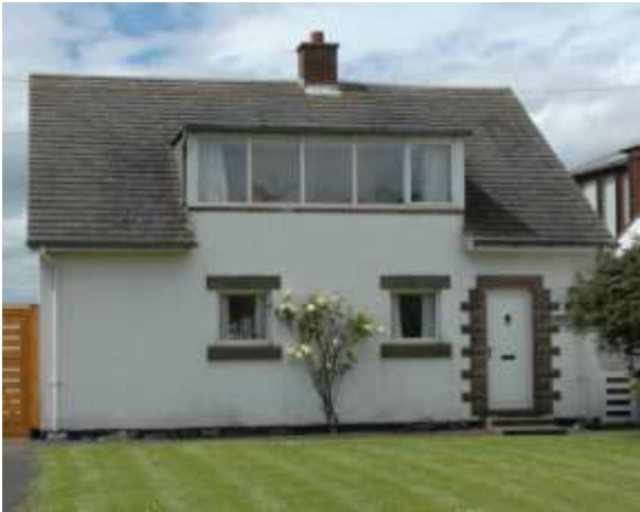
An interesting design with hint of Arts and Crafts. There is still plenty of roof slope visible
