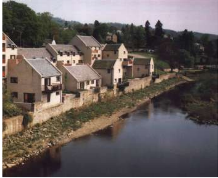
High density new housing near Perth
