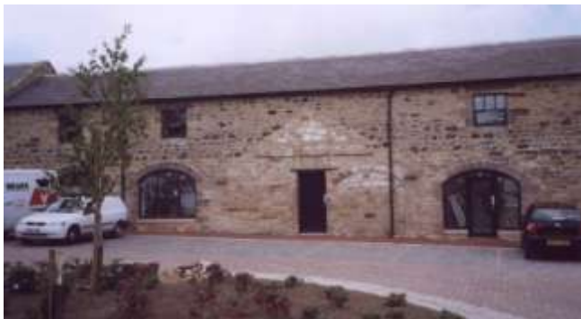
Conversion of farm buildings into workshops and office space at Hawkhill Farm.
